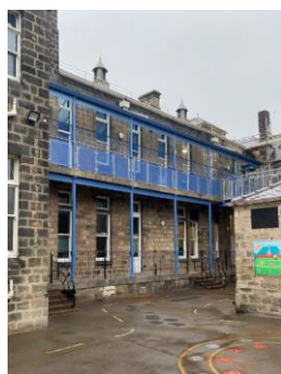
Removal of external fire escapes and complete replacement of balcony metal work.
